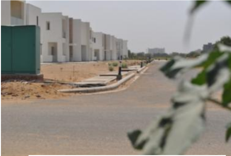
Cluster of houses connected to STP
