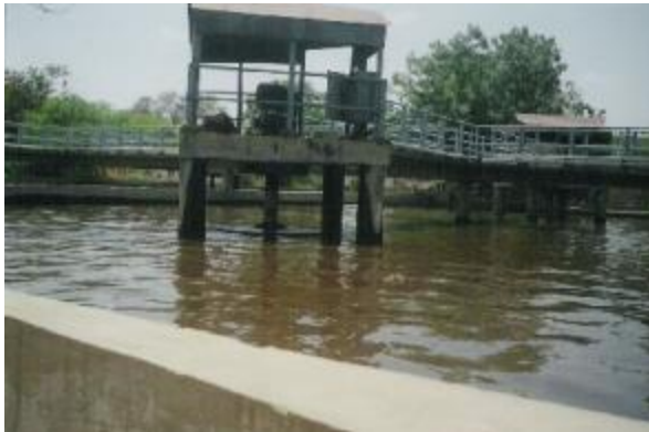
Aerators being turned off
