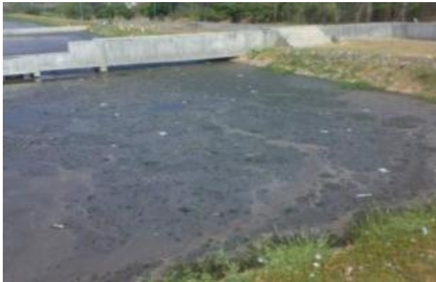
Sludge deposits in sewage
