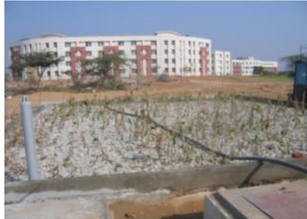
Gravel Plant Filter
